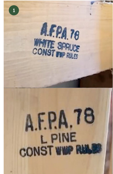
1. Examples of grade stamps first used under the Western Wood Products Association standards. The grade stamp shows construction grade white spruce and lodgepole pine, using WWP rules. A.F.P.A. 78 is the identifier for the now inactive Nelson Lumber.
